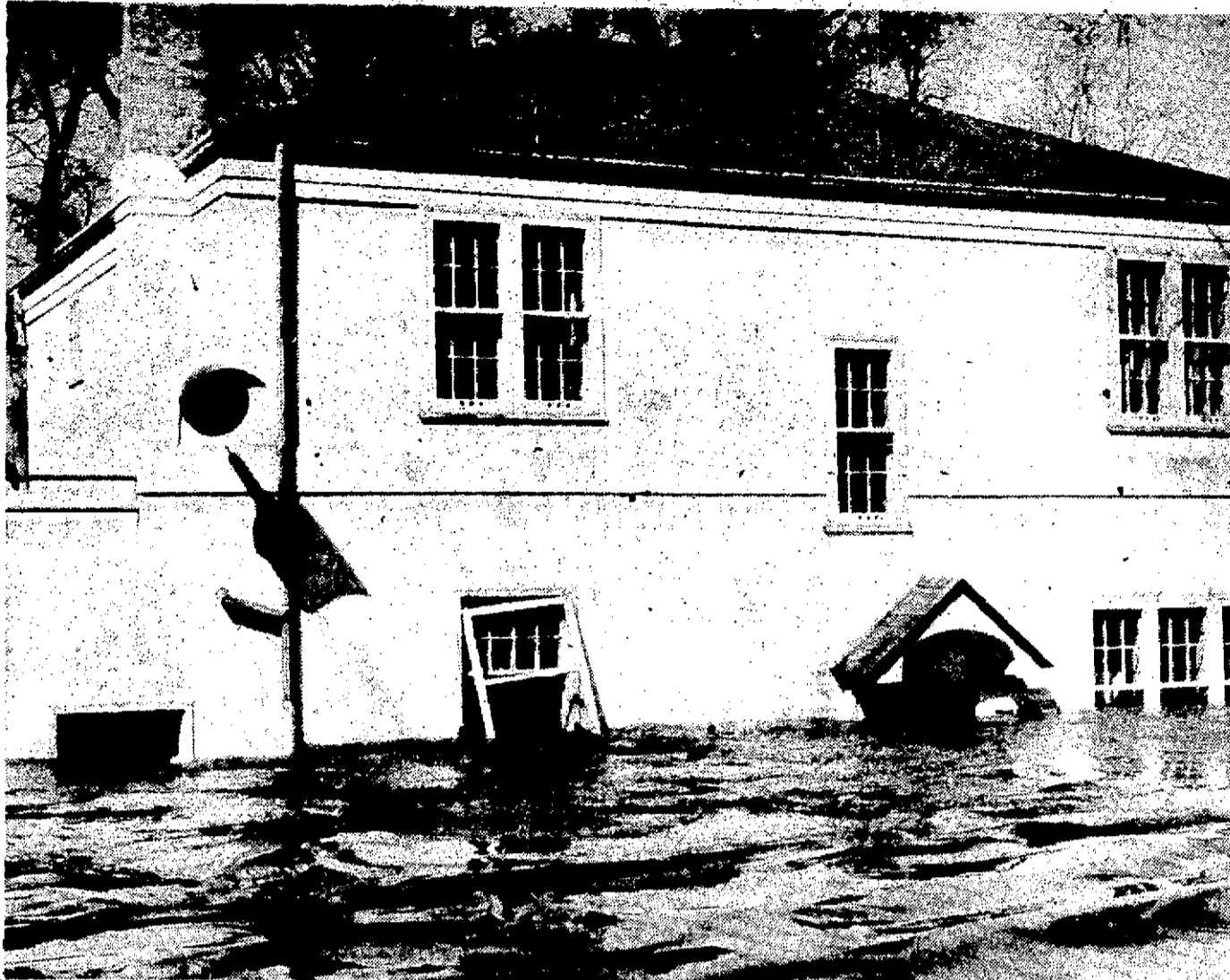
Water is almost up to the second storey of this house located on the south side of Elm Park. The door and windows have been left open.
