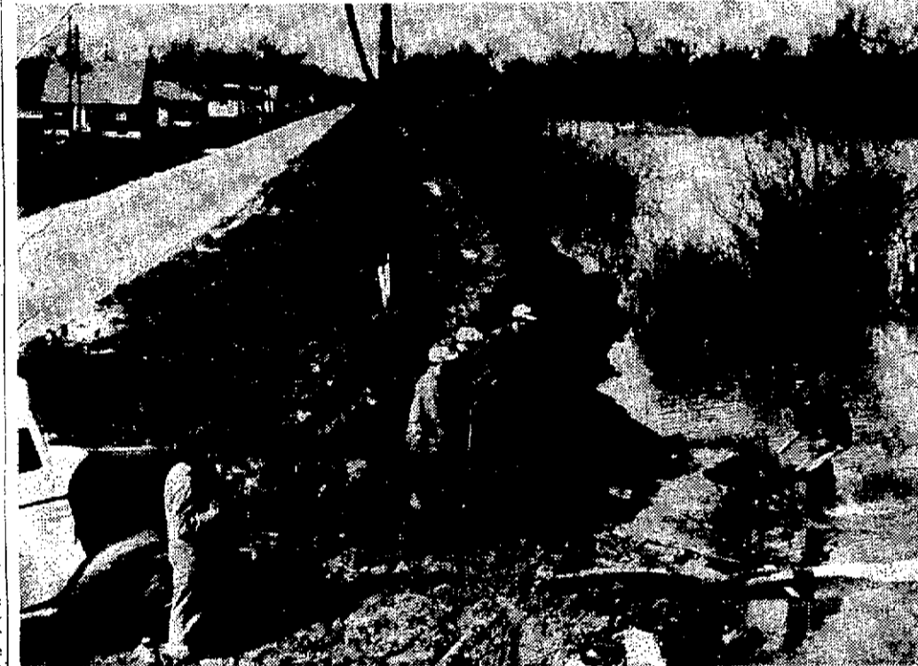
This giant dirt dike running southwest along Oakenwald avenue, Wildwood, is holding back five feet of water.
