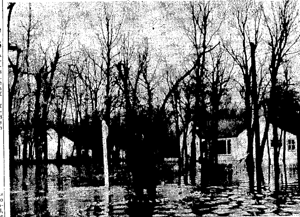
Flood water rising to this level around many Victoria crescent, St. Vital homes, has forced evacuation of about 20 families.
