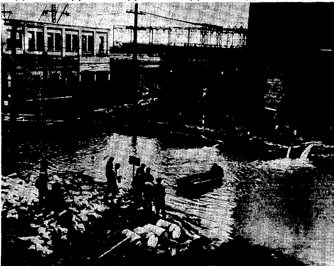
Essential to the winning of the flood battle is complete maintenance of power feeder lines throughout the city and right in the front line of the river's attack is the Mill street sub-station (above) where service men and volunteers are fighting a ceaseless war against the rising water. Dikes, heavy duty pumps and other flood-fighting equipment are being used to protect vital dynamos and transmission circuits.
