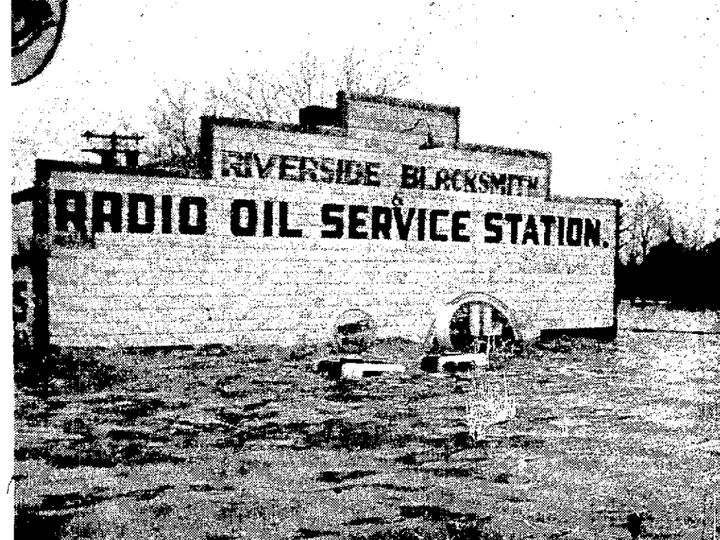
A service station at Morris surrounded by water several feet high.
